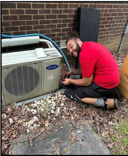
William Swan, WJCC student, HVAC Intern, assisting HVAC in performing preventative maintenance.
