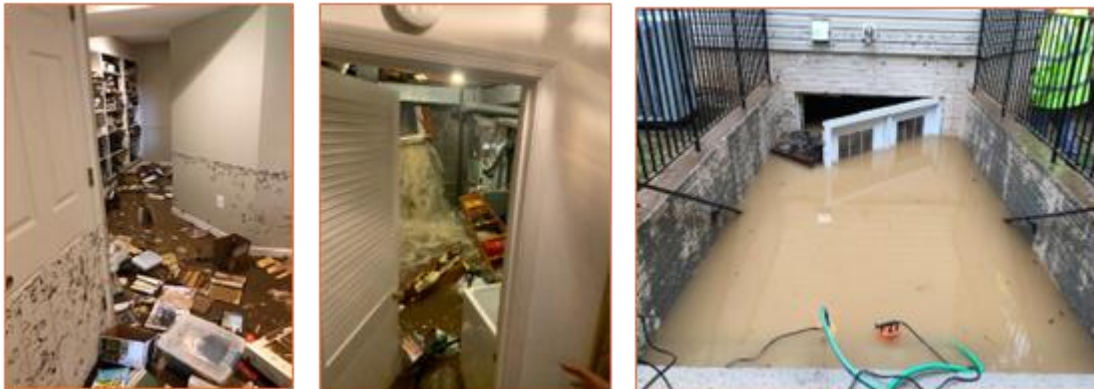
Figure. Photos of damage to residential property from flooding in July 2019
