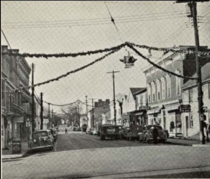
LOOKING SOUTHWEST ON MAIN STREET
