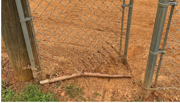
Broken fencing was frequently curling up at ground level, presenting a hazard to play.
