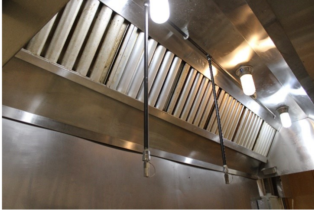
A new fire suppression system increases safety and allows concession stand use.
