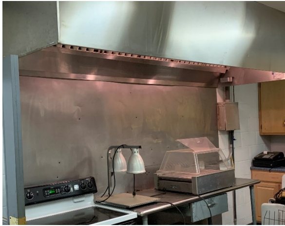
The concession stand hood lacked any fire suppression system, and was not safe to use.
