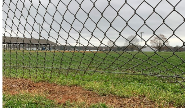
Broken fencing was frequently curling up at ground level, presenting a hazard to play.
