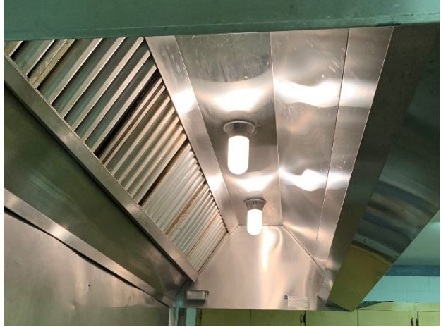
The concession stand hood lacked any fire suppression system, and was not safe to use.
