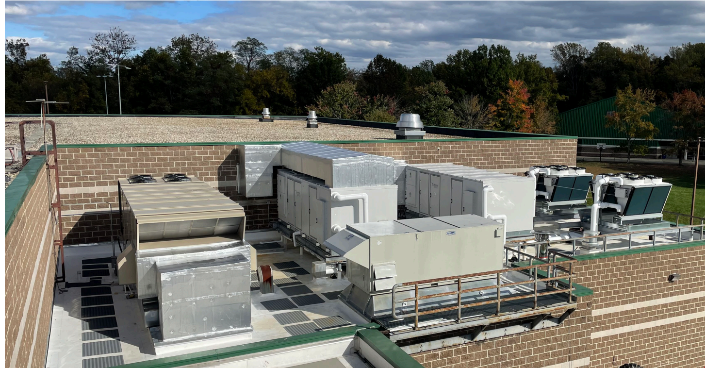
South Run Rec Air Handlers and Pool Dehumidification Units
