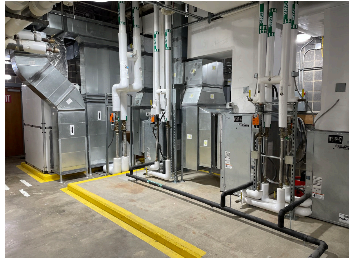
Spring Hill Rec Center DOAS and WSHPs
