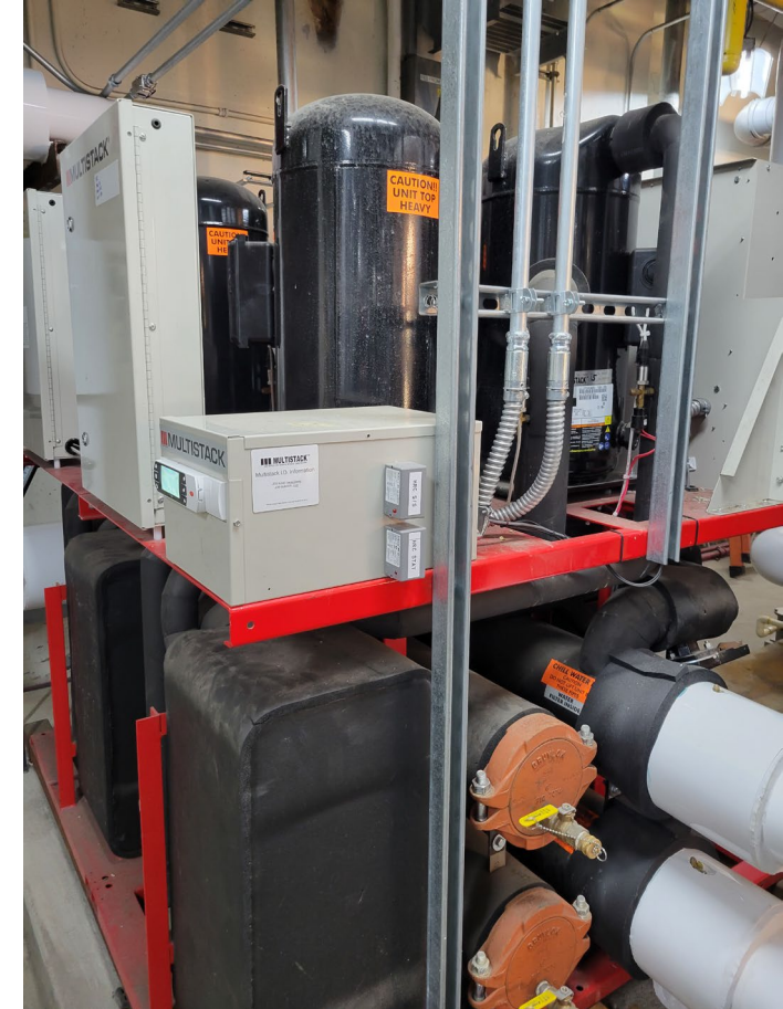
Cub Run Rec Pool Heat Recovery Chiller
