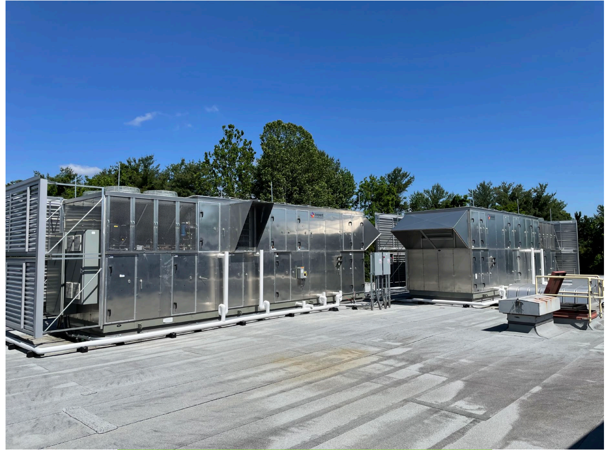
Spring Hill Rec Pool Dehumidification Units
