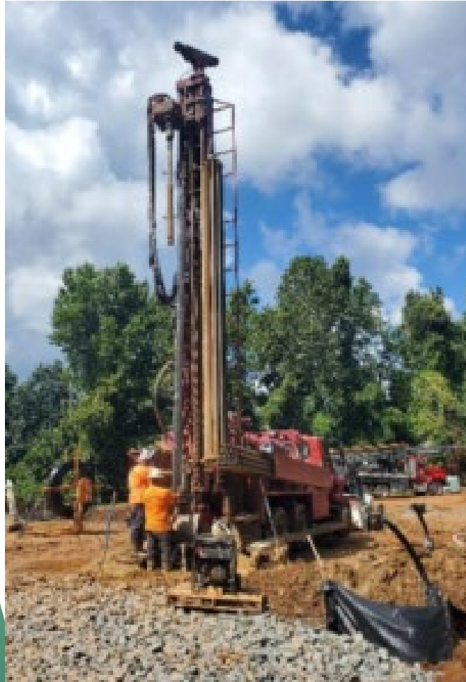
Spring Hill Rec Center Geothermal Wellfield
