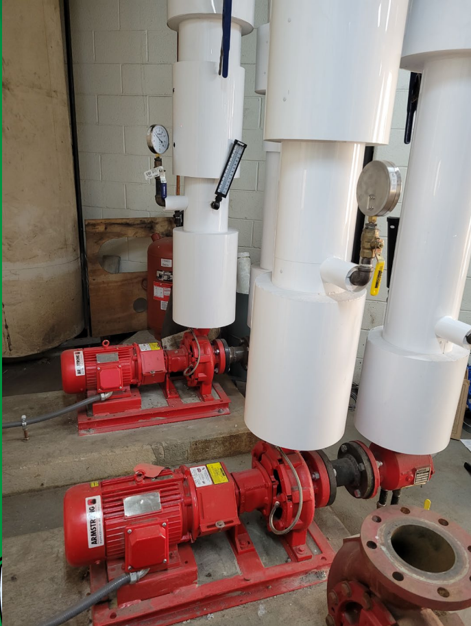
Cub Run Rec Heated Water Pumps
