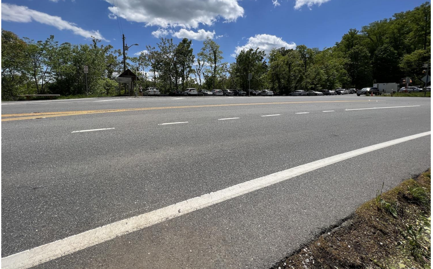
A pedestrian bridge is coming, but for now hikers must cross busy Route 311 to get to the McAfee Knob trailhead/Jennifer Bain
