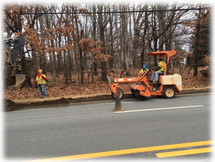
VDOT Street Sweeping 12 miles of Route 29 Business
