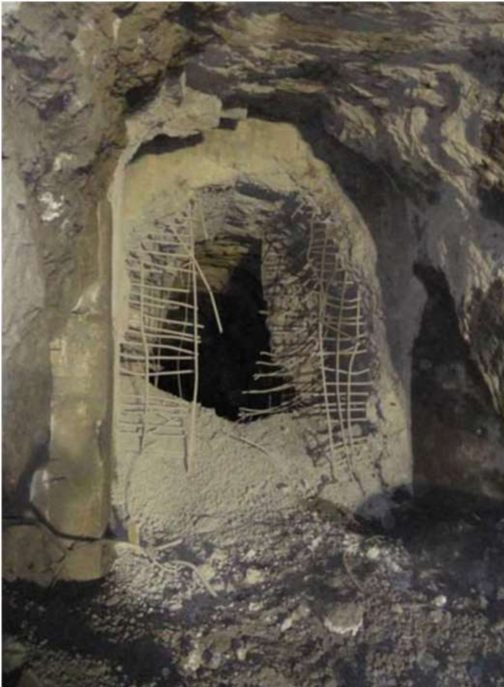
Looking at the eastern bulkhead that was blocking access within the interior of the tunnel after fourth blast. This proved to be a more challenging operation than originally anticipated. Photo courtesy of VDOT.
