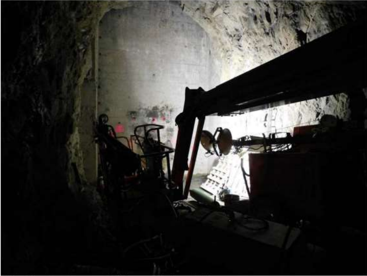
Drilling blastholes in east seal. Drill set up on basket of hi-lift.
