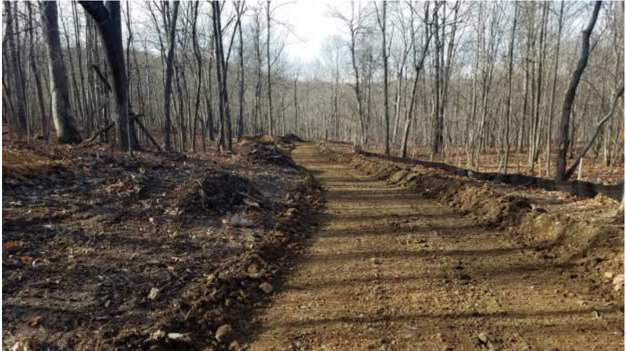
Grading of western trail. Photo courtesy of Woolpert Inc.
