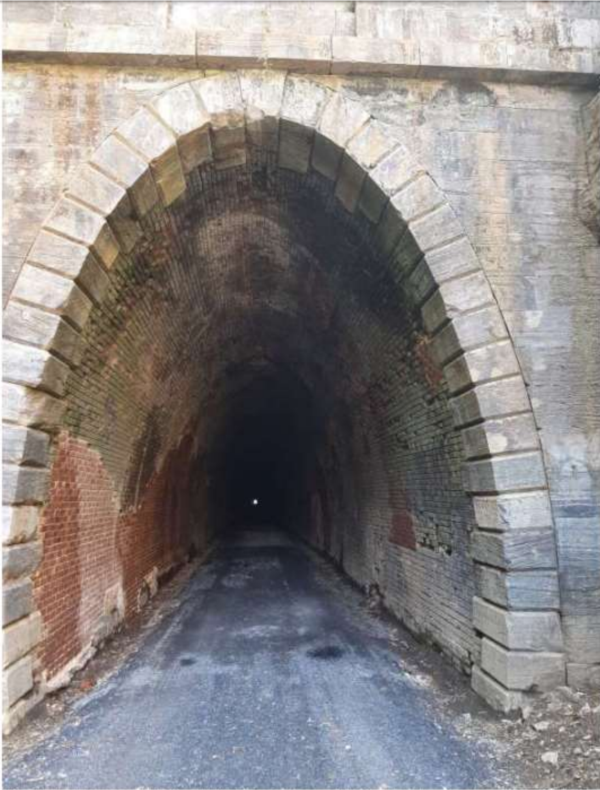
"The Light at the End of the Tunnel." We have been waiting for this view for many years! Note the repaired/replaced brick masonry units and surfaces scrubbed of decades of graffiti, as well as the new drained trail bed.
