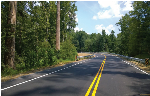
VDOT Route 651 Highway Project, Hanover County, VA
