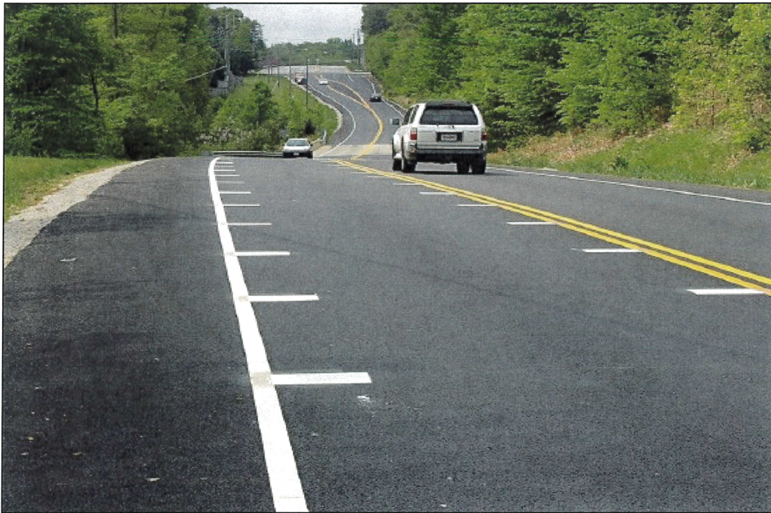
Figure 6: Proposed Innovative Solutions to Reduce Speeding – Optical/Speed Bars
