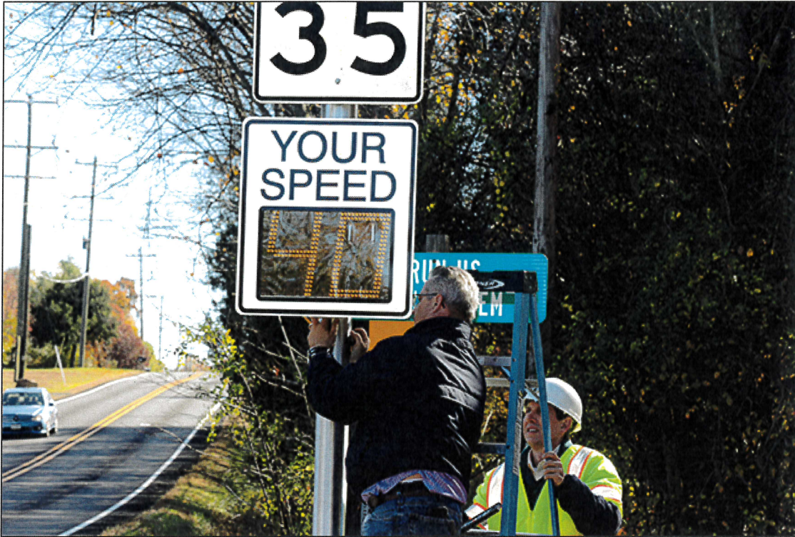
Figure 5: Pole-Mounted Speed Display Sign
