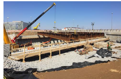
Jones Branch Connector Bridge
