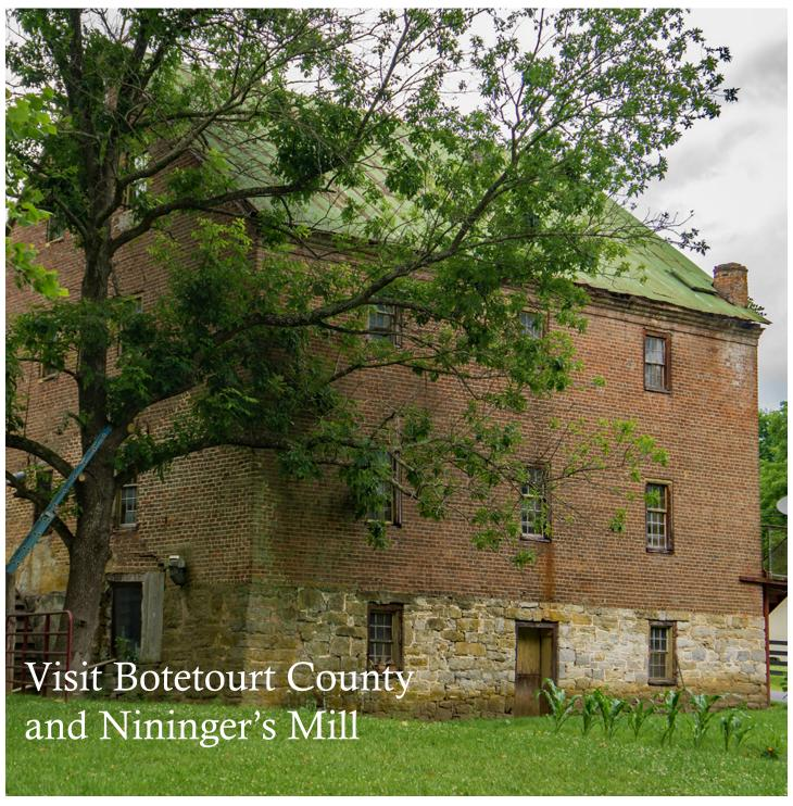
Nininger's Mill, also known as Tinker Mill, is a historic grist mill located near Daleville, Botetourt County, Virginia. The mill was built about 1847, and is a three-story, brick structure with a gable roof. Wood-frame additions added in the 20th century, are found on the north and east walls. Also on the property is a contributing simple one-story, wood-frame late 19th-century house. The mill was converted to restaurant in 1980.
