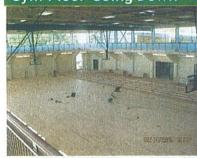
This picture shows the gym floor being installed this week. Our floating wood floor features a double layer of solid wood with cushioned shock absorbing pads. That means playing basketball or working out on this surface will be easier on the joints.
