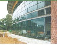
The last windows are being installed at Green Ridge next to the indoor pool. Even though the building will contain a large amount of glass, it's specially designed and tinted to reduce energy loss from heat transfer. That's one of the many
