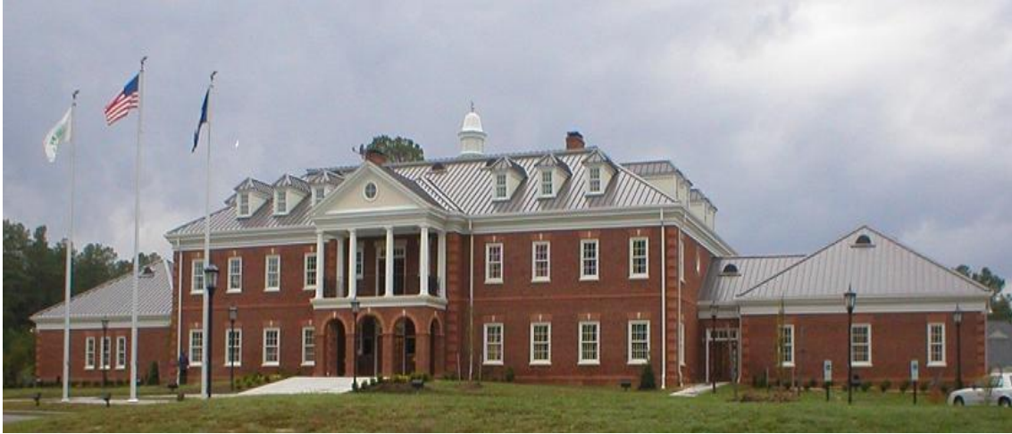
Greenville County Government Building
