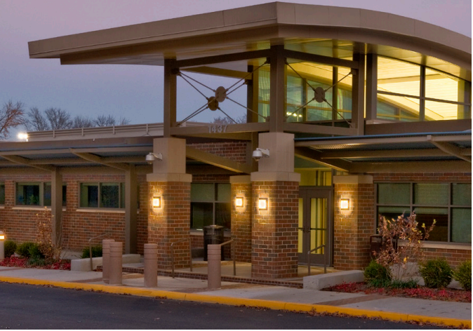
McLean District Police Station and Governmental Center Renovation and Addition, Fairfax County, VA
