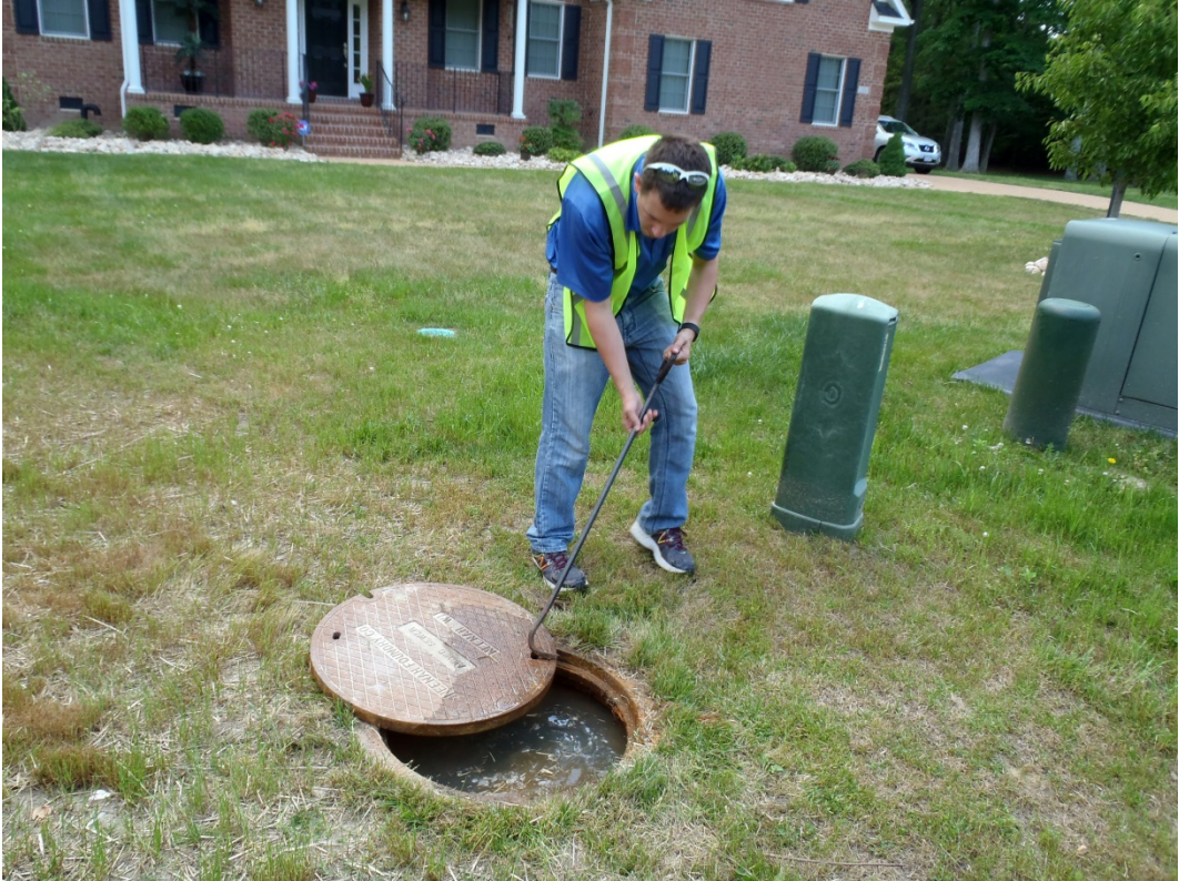
Photo shows vacuum pit full of water and proximity to residence.
