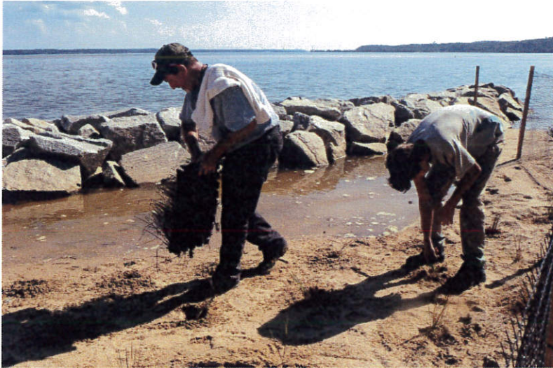
Planting the wetland marsh behind each sill
