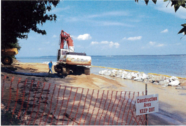
Living Shoreline under construction
