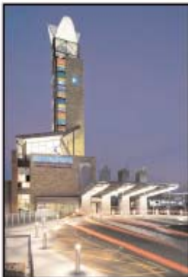
Dell Children's Medical Center of Central Texas - First healthcare facility in the world to receive LEED Platinum Certification.
